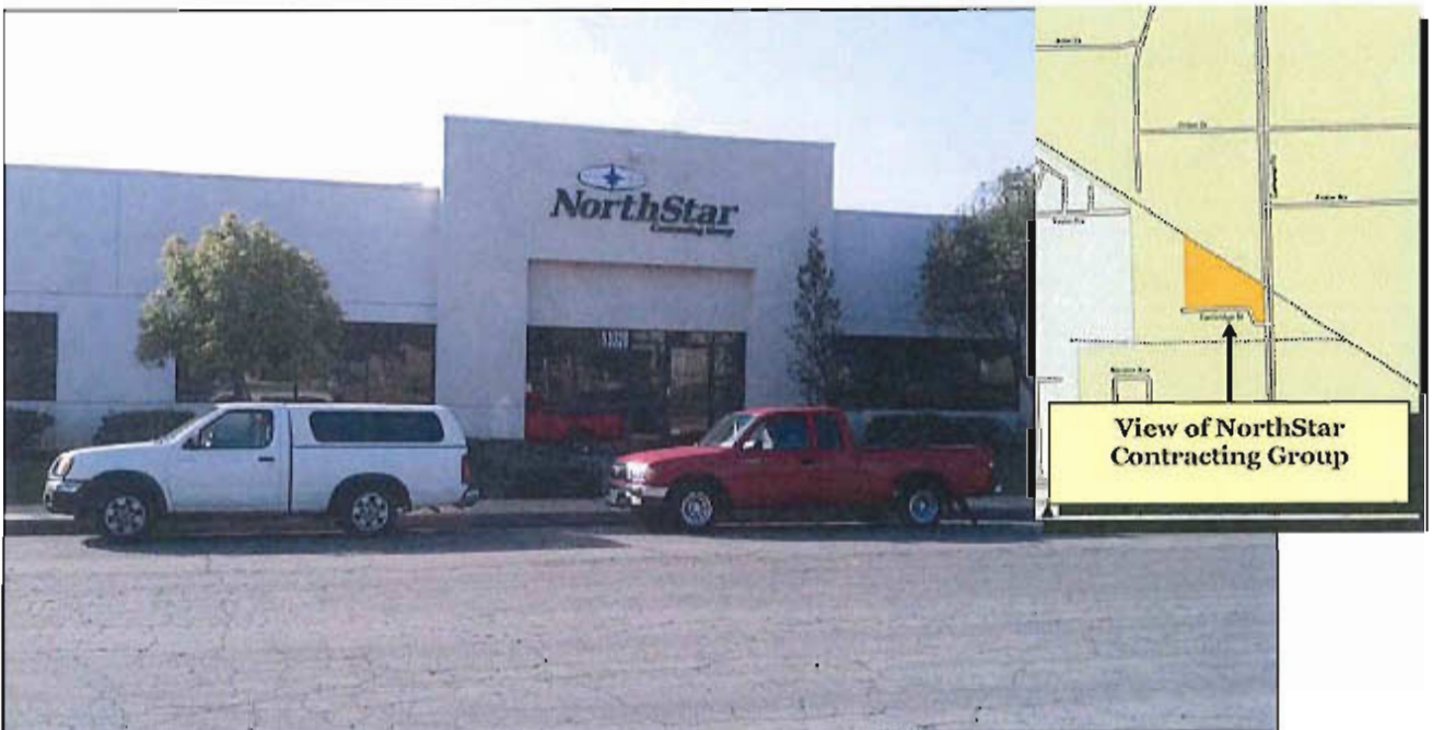
View of the existing NorthStar Contracting Group facing south
