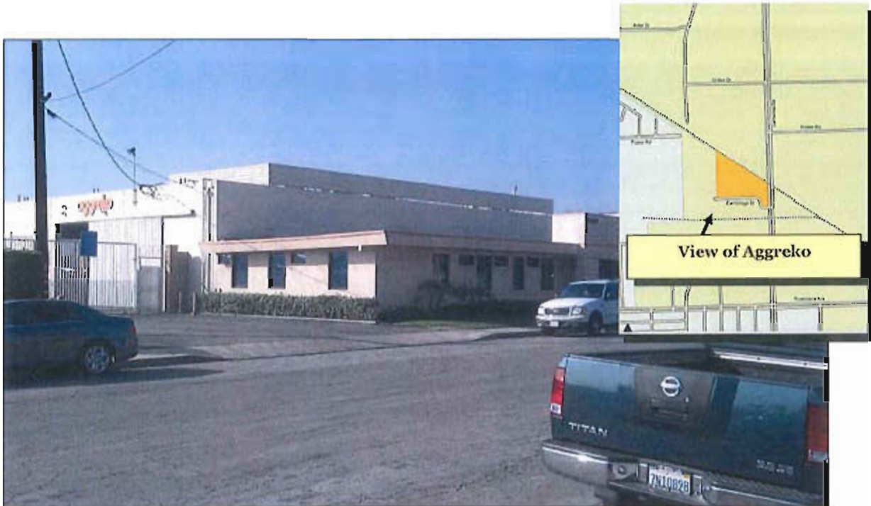
View of the existing Aggreko facility facing southwest
