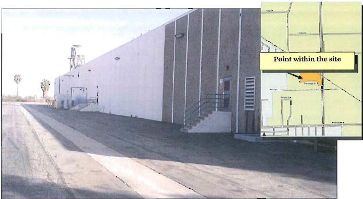
View of the existing concrete tilt-up structure and drive aisle facing northeast
